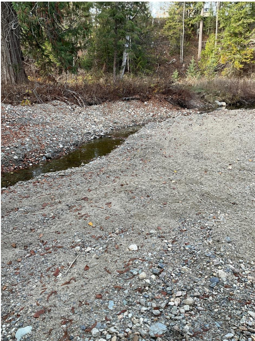
Figure 5. Gravel placement appears to have been placed to block a side channel and machinery tracks are visible instream (left). Riparian vegetation has been cleared, and bed material has been excavated along a property at the end of Creekside Road.
