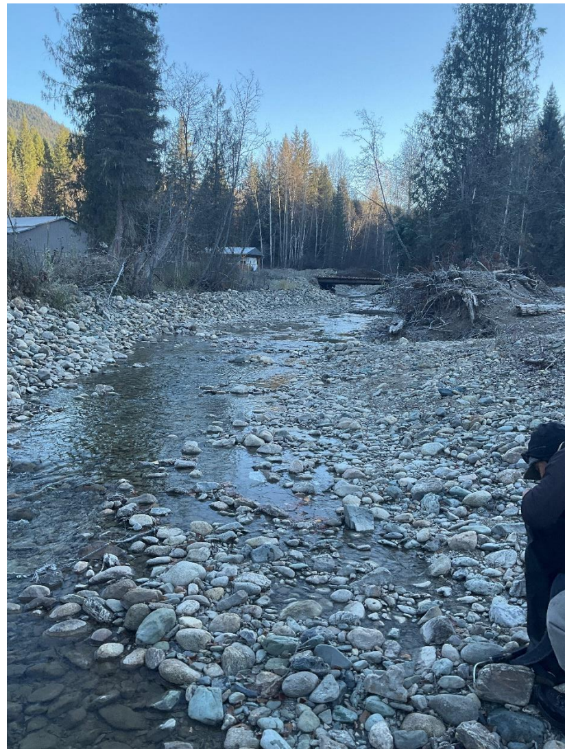
Figure 5. Gravel placement appears to have been placed to block a side channel and machinery tracks are visible instream (left). Riparian vegetation has been cleared, and bed material has been excavated along a property at the end of Creekside Road.
