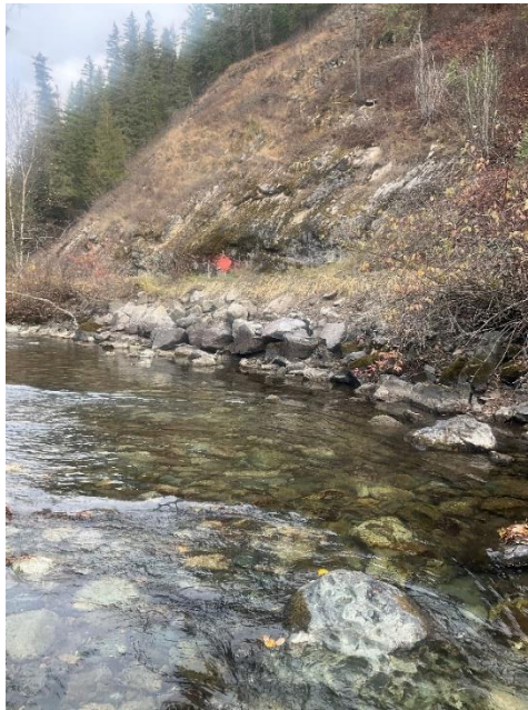
Figure 17. A long section of riprap along the road confines the stream. The banks are too steep for vegetation and are sloughing road material into the creek.
