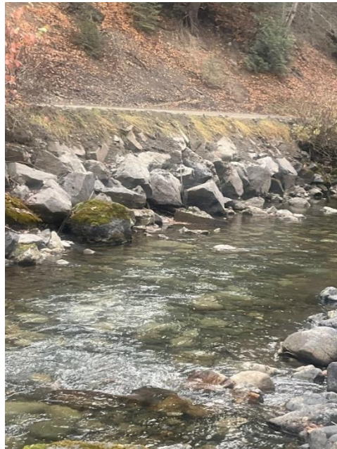
Figure 17. A long section of riprap along the road confines the stream. The banks are too steep for vegetation and are sloughing road material into the creek.
